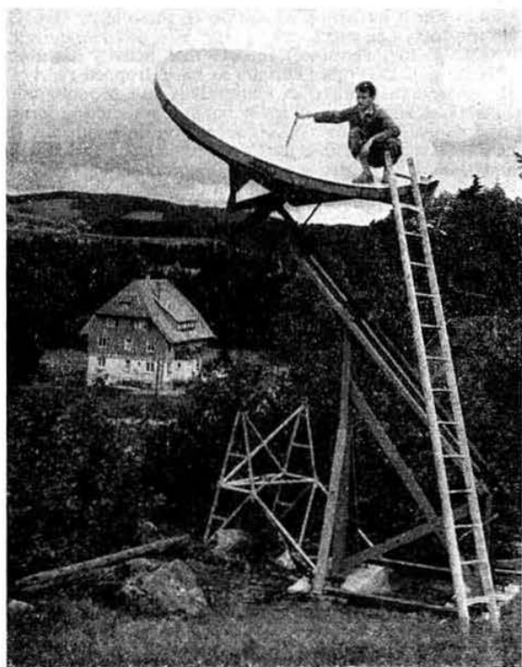
DJ3EN adjusting his 15 ft. dish aerial for moon-bounce experiments
